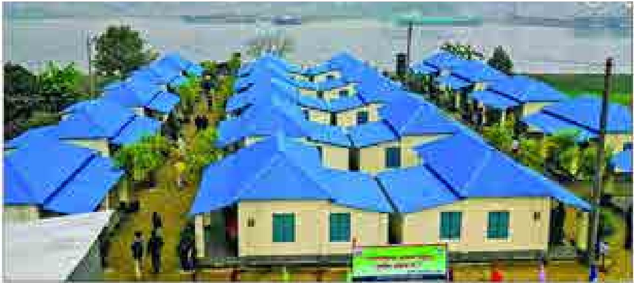
A portion of houses built for destitute people in Bangladesh under the Ashrayan Project.
