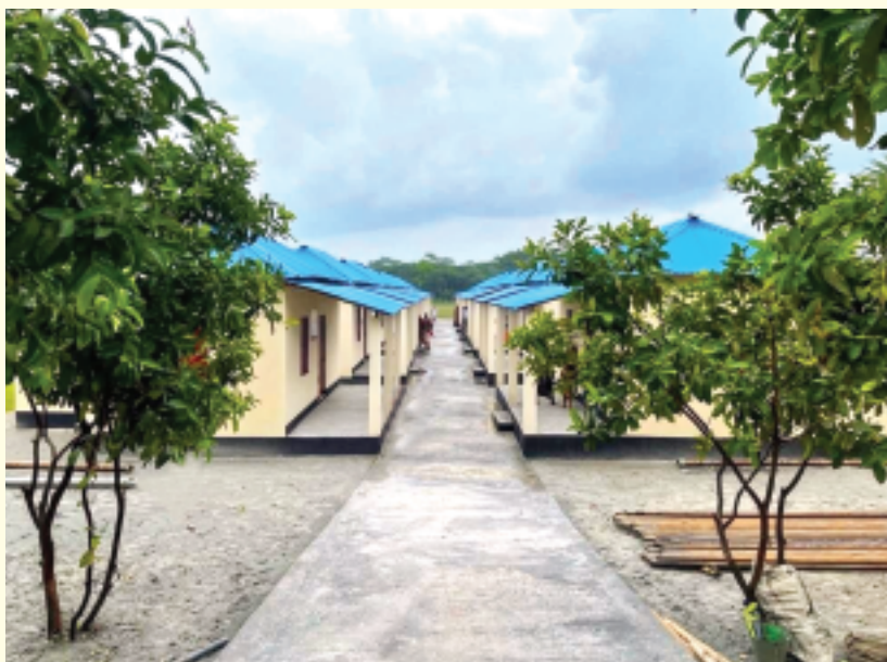
Internal road in a project area
